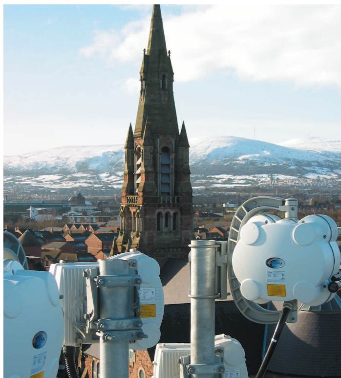
The Belfast network uses SONAbeam optical transceivers and 802.11b radios.
