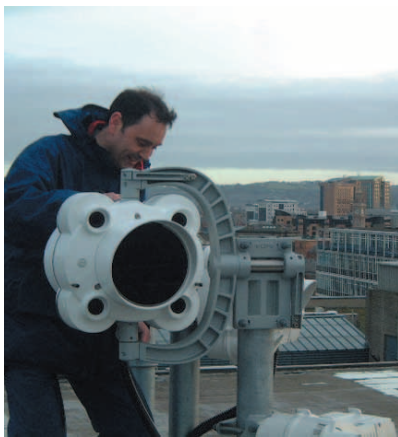
SONAbeam installation for the Flax Trust network.
